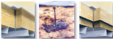
Corrosion of fastening elements in flat roof applications will occur; specifically with wet or damaged substrates.
